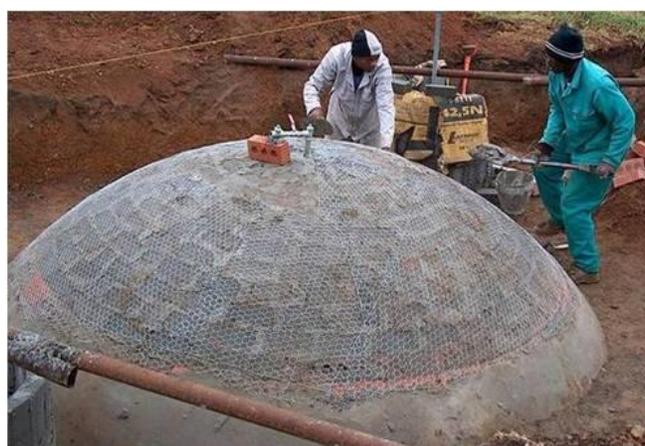
Figure 18. Fixed Dome Digester During Construction
