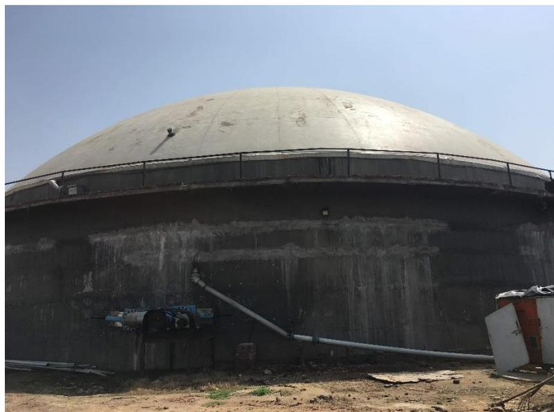
Figure 24. Completely Mixed Digester
