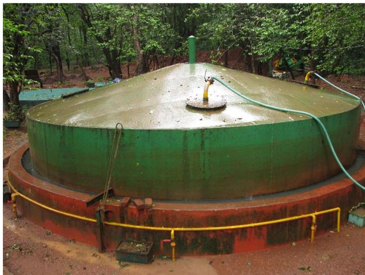
Figure 22. Floating Drum Digester
